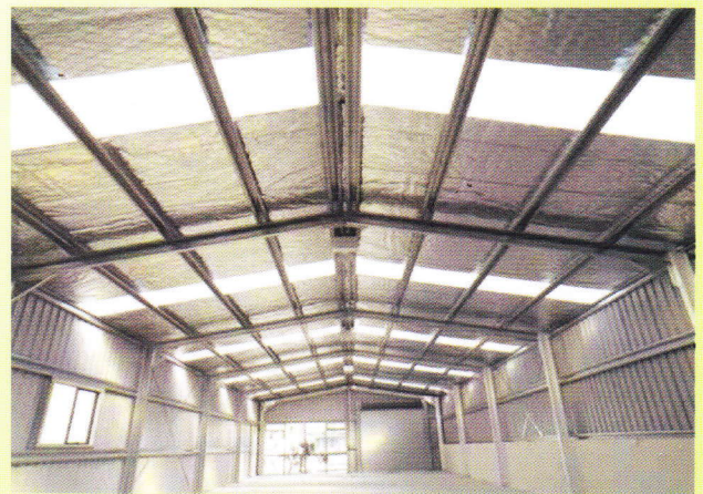
Batten used in portal frame warehouses as alternative to Z / C Channel Section
